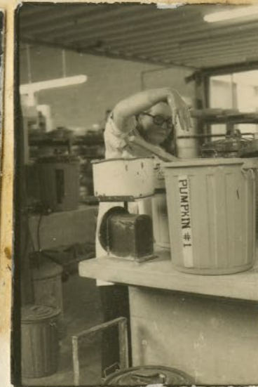
A PROBLEM WITH A GLAZE - CHECKING SPECIFIC GRAVITY AND VISCOSITY -
