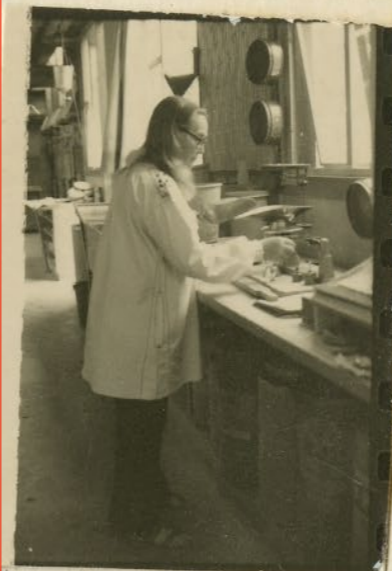
A PROBLEM WITH A GLAZE - CHECKING SPECIFIC GRAVITY AND VISCOSITY -
